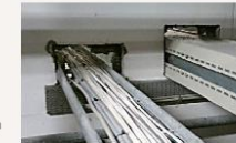
Picture shows an example of unsealed penetrations through a fire rated wall.
